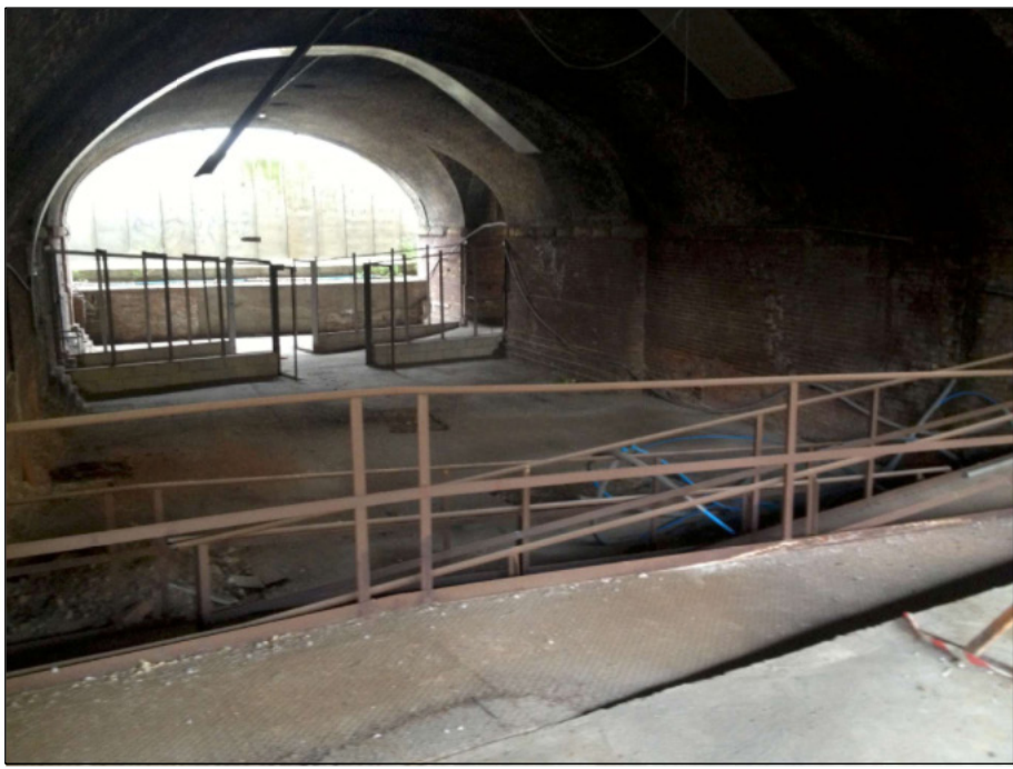
EXAMPLES OF VARIATION IN FLOOR LEVEL AND FINISH - Existing condition to be excavated/filled to facilitate level access to all areas from London Road.
